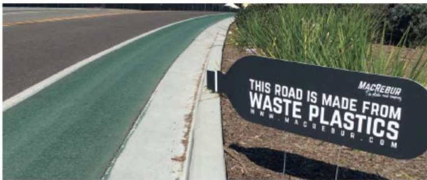
▲ Figure 20.28 Plasphalt is made up of grains of plastic produced from unsorted plastic waste. This replaces the sand and gravel usually used in asphalt production for road surfaces. It can also contain recycled glass pellets
